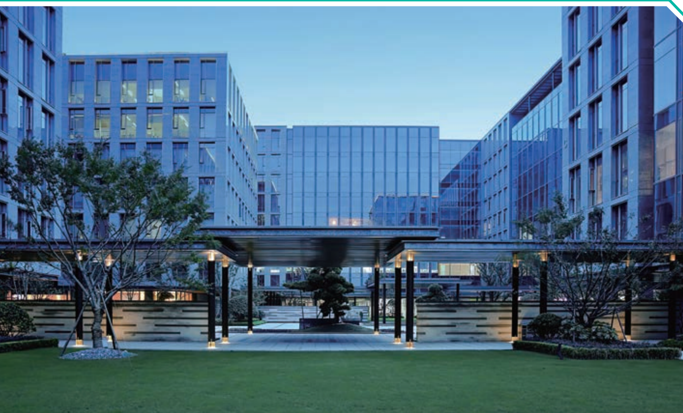
Greentown Management Headquarter (Greentown • Hangzhou Xixi International)
