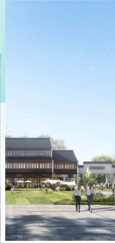
Neighbourhood centre: Zhoushan New Port Project
