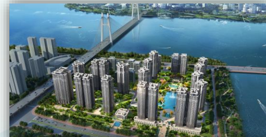
Guangzhou Nansha Project (AVIC Trust)
