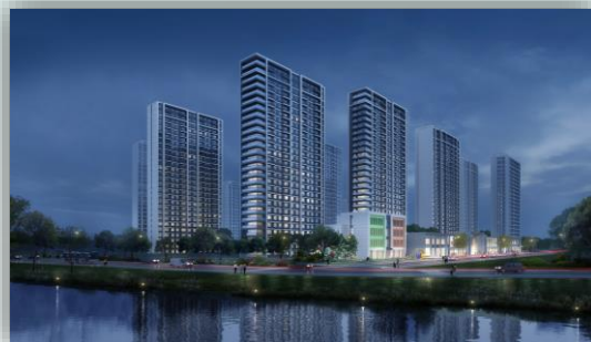
Changchun Erdao Riverside Project
