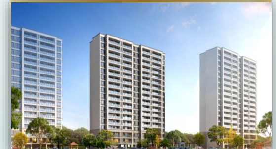
Wuxi Jiangyin Yunting Street Project
