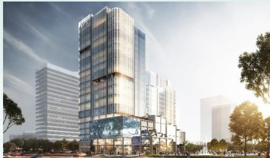
Hangzhou Chenfan Headquarters Building Project (Live Broadcast Base)
