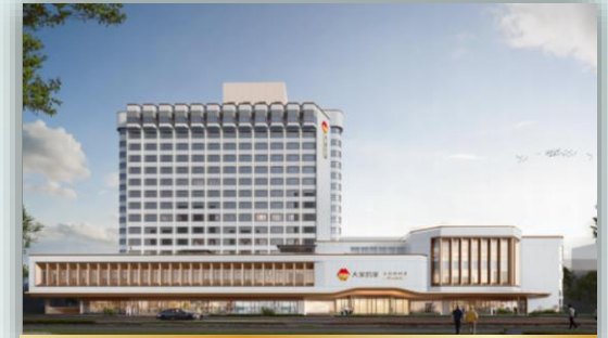
Hefei Wutongli City Center Community Renovation Project (Community Renovation)
