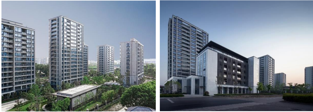
Image: Jinhua Qinjian Yaju Affordable Housing Project
