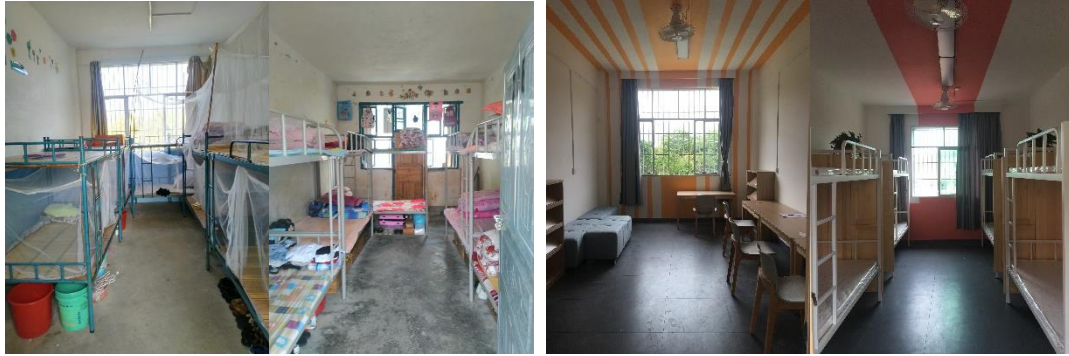
Image: Before and after the renovation of the school building of Xunwu Rural School in Jiangxi
