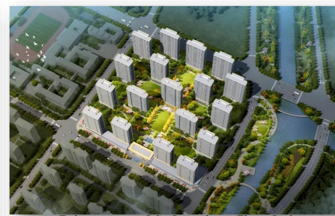
Joint-ownership housing: Jiangbei District Project in Ningbo City
