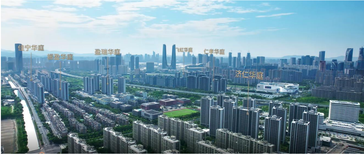
(Image: Qianjiang Century City Resettlement Housing Project)
