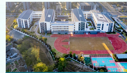
Hangzhou Binjiang Zhenpu Primary School
