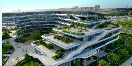
Iflytek Industrial Office Project
